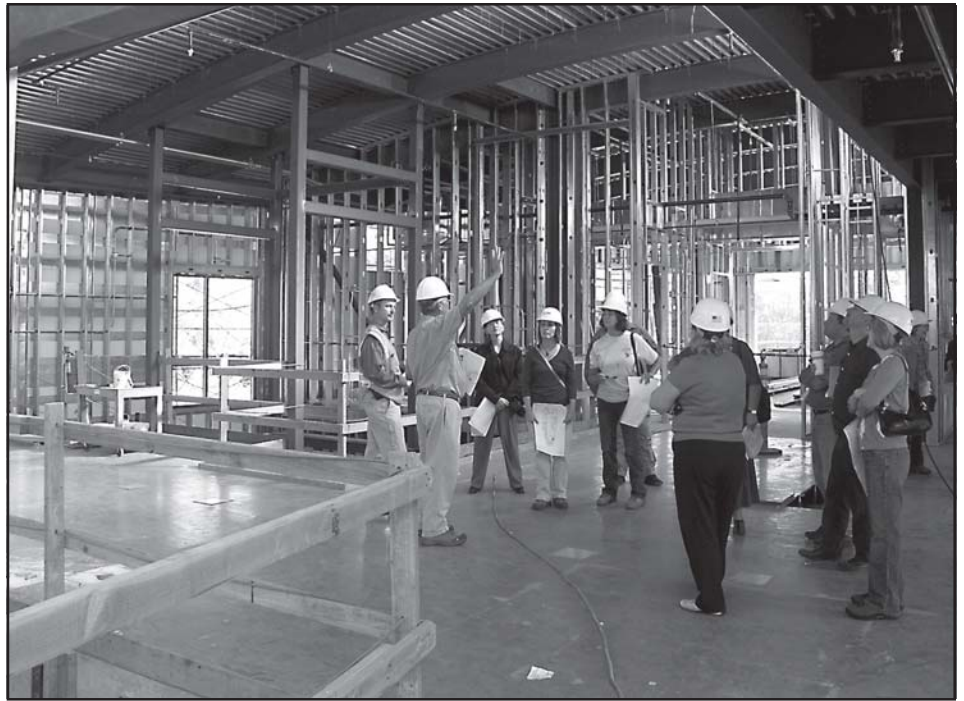
GROWING A GREEN LIBRARY — Walnut Creek Library Foundation Steering Committee Member Bob Brittain explains the "daylight harvesting" feature of the new downtown library to a group of library staff. "Daylight harvesting" means the lights automatically dim when bright sunshine comes through the window, reducing energy use. Green practices such as this are among the reasons the new library will be LEED certified, the recognized standard for building sustainability. Construction of the new Walnut Creek Library continues on time and on budget with a planned opening in mid-2010.
